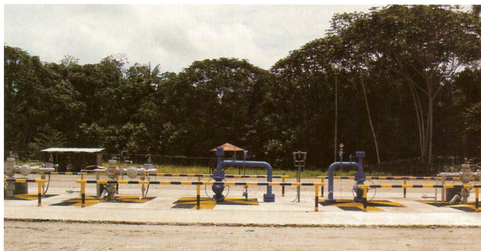
Figure 6: Wastewater reinjection pumps.
