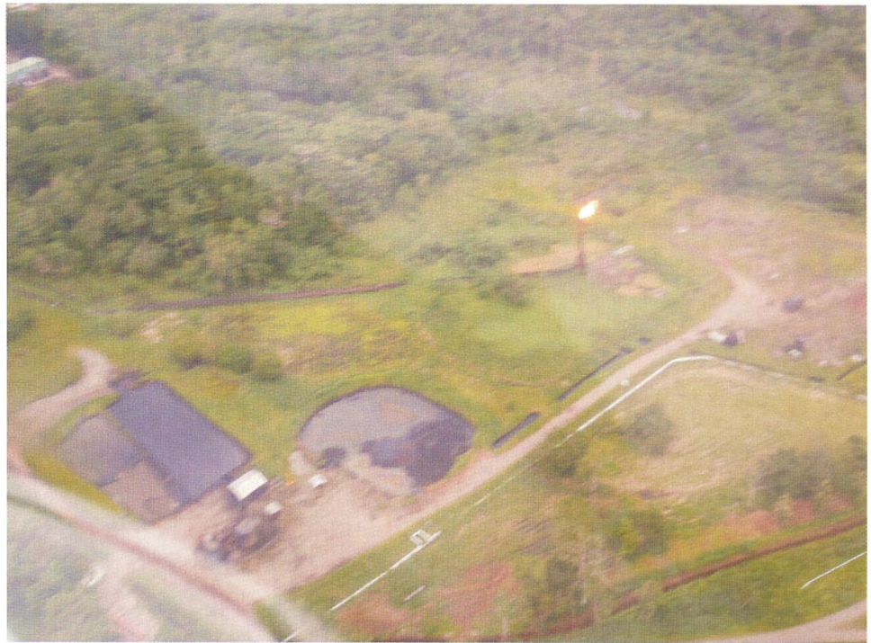
Figure 14: Open oil pits and gas burner.
