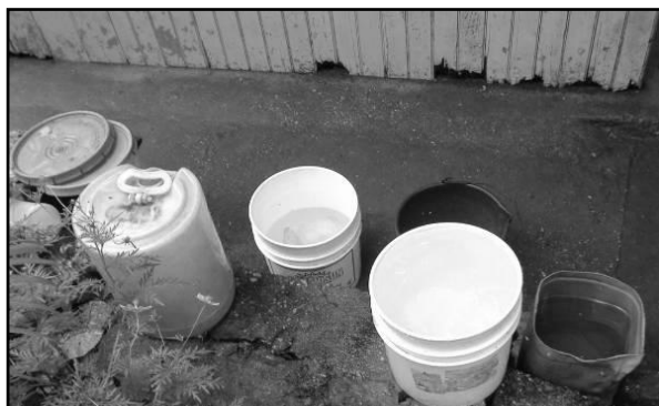
Figure 6: Buckets aligning the roof line to catch rainwater.
