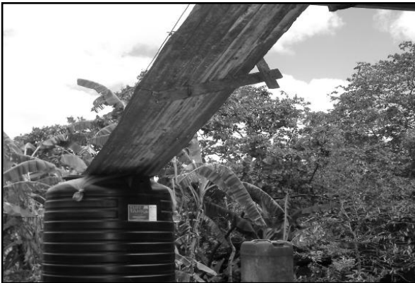
Figure 5: Rainwater collection from the roof to buckets and tanks.
